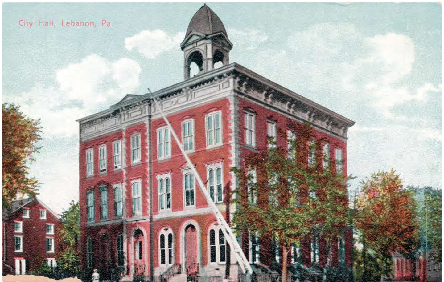
Lebanon City Hall Building with a raised railroad crossing gate – postcard - ca. 1912. Source-Randy Jaye collection.
