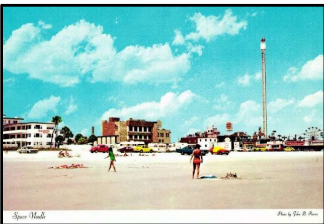
Daytona Beach's Space Needle. Postcard ca. 1970. Author's collection. Note: In 2012, it was demolished after becoming structurally hazardous and deemed an eyesore.
