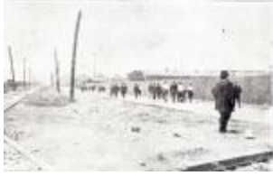
Wall surrounding the Pressed Steel Car plant, McKees Rocks, PA, 1909.
