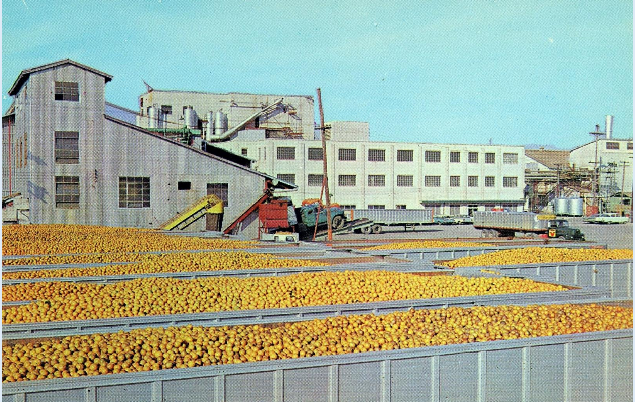
Minute Maid Processing Plant - Florida - ca. 1950s.
