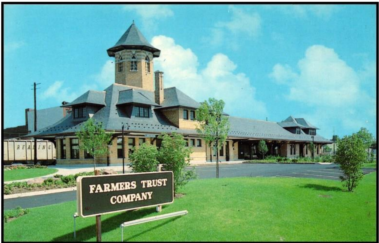
Postcard showing the restored and repurposed Philadelphia & Reading Railroad Station in Lebanon, circa 1979. The railroad station was used by the Farmers Trust Company from 1977 to 2002. (Author's collection)
