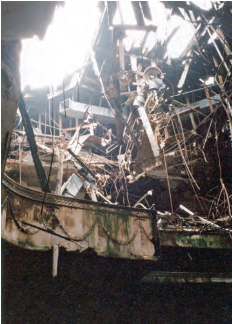
Colonial Theatre - The hole in the roof Summer 1996. Courtesy of Hillary Hess
