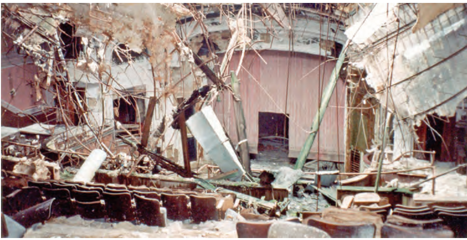
Colonial Theatre - A view from the balcony looking toward the stage - the roof had collapsed Summer 1996 - Courtesy of Hillary Hess
