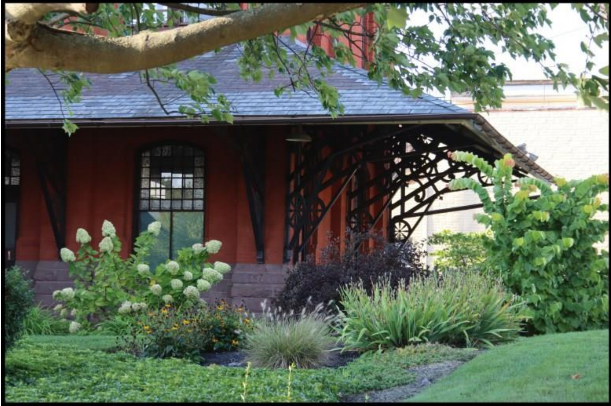
Southeast view of the Cornwall & Lebanon Railroad Station in 2022, with focus on the ornate iron roof brackets. (Randy Jaye)
