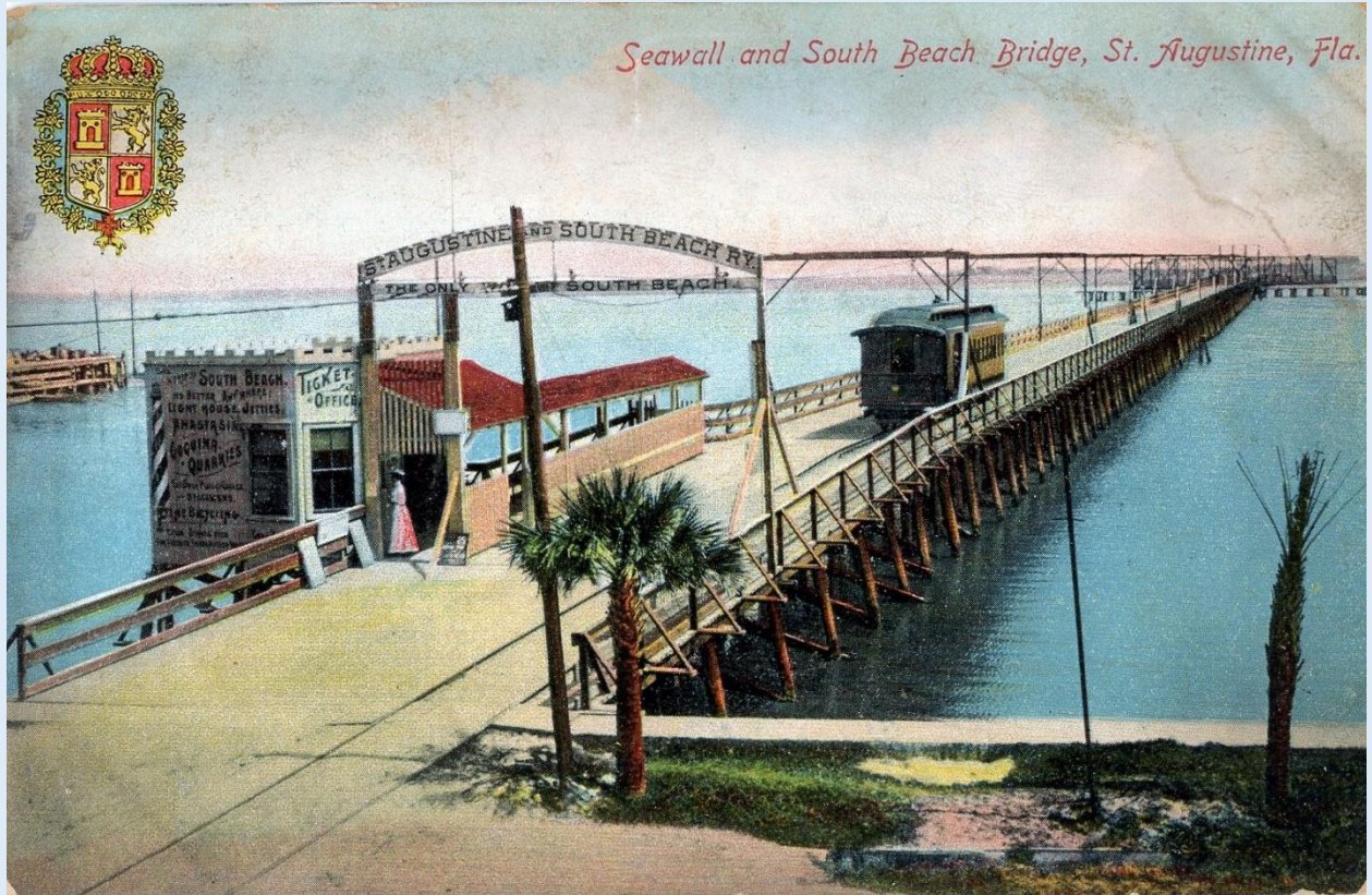
Sea Wall and South Beach Bridge - St. Augustine, Fla. - ca. 1920s.
