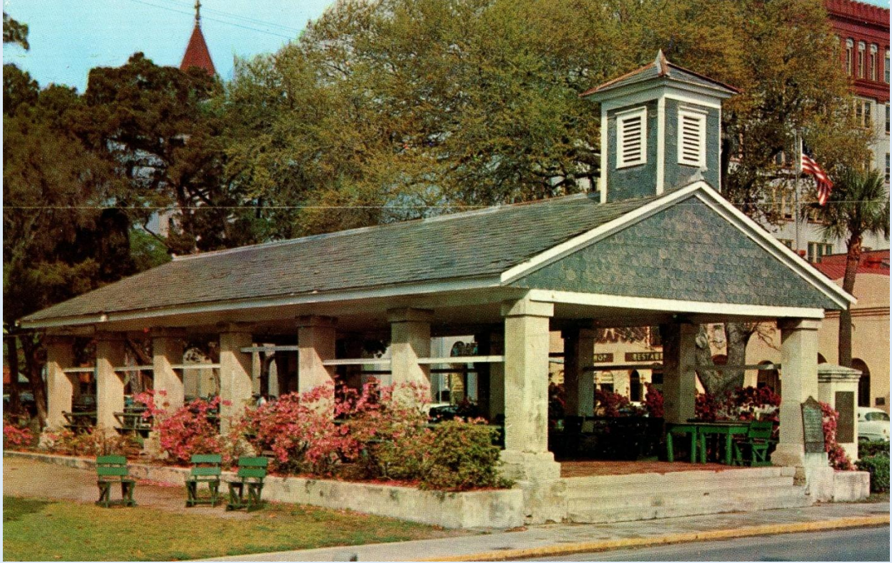
The Old Market - this structure dates from 1824 - St. Augustine, Fla. - ca. 1950s.
