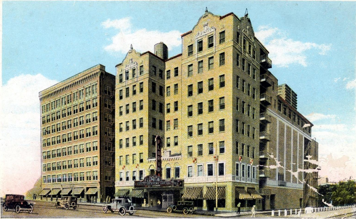
FLORIDA THEATRE BLDG., AND FIRST NATIONAL BANK.
