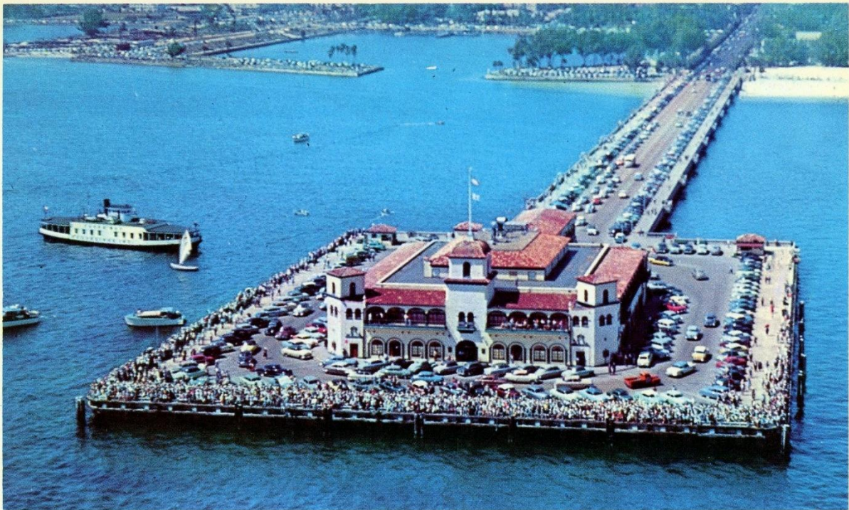
Municipal Recreation Pier, St. Petersburg, Florida
