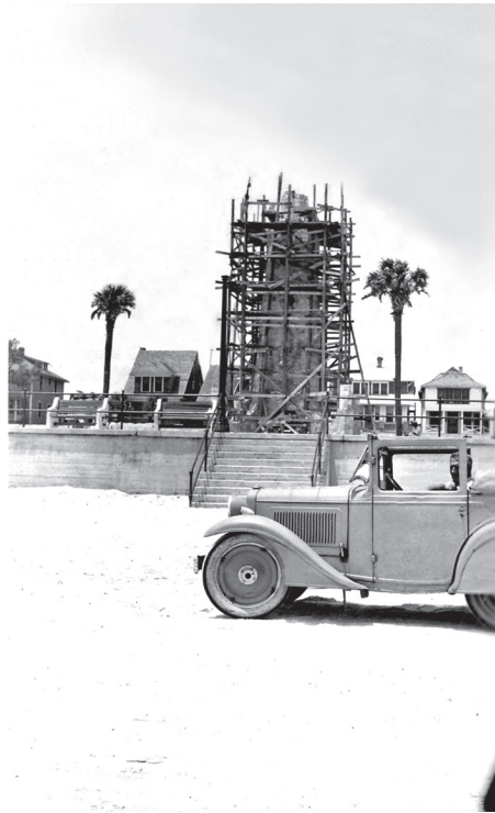
Figure 5. Under construction, circa 1937. The base, body, and cupola are complete. A curious WPA worker sits in a construction vehicle on the beach. PHOTO COURTESY OF THE HALIFAX HISTORICAL MUSEUM.
