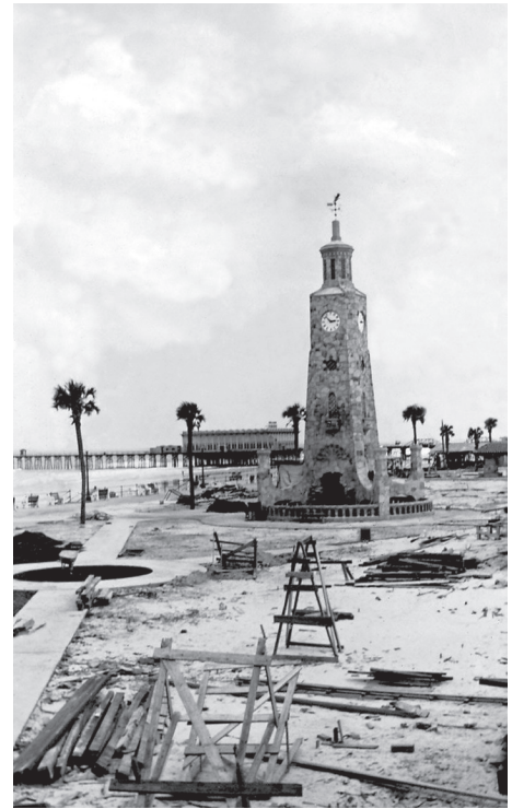
Figure 6. Construction nearing completion, circa 1937. The scaffolding lumber and tools are in the process of being removed from the construction site. PHOTO COURTESY OF THE HALIFAX HISTORICAL MUSEUM.
