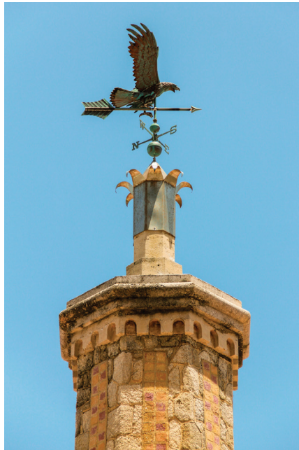
Figure 9. Stainless steel base cap with decorative petals and weather vane. Photographed by Randy Jaye on August 5, 2015. (Note: This stainless steel cap was removed in March 2016 when a period-correct concrete Spire was constructed.)
