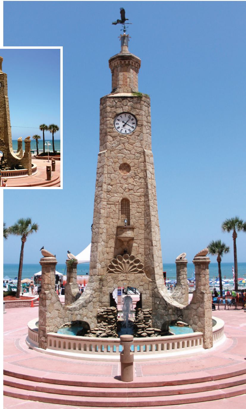
Figure 2. The clock tower (photographed by Randy Jaye on August 5, 2015) had a non-original petal base (stainless steel base cap) with decorative petals and a non-original but period-correct, copper-sheathed eagle weather vane.
