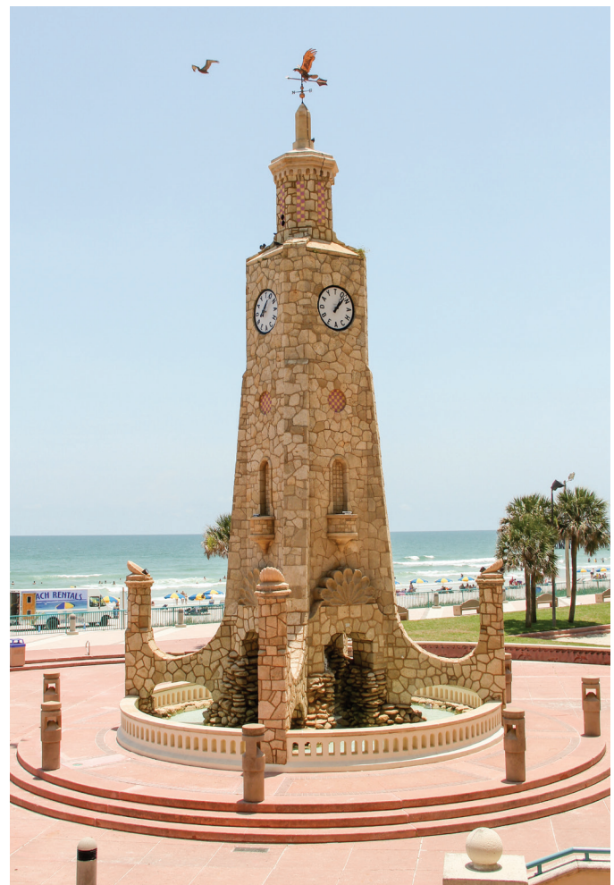
Figure 16. The clock tower's new look after the completed 2015–2016 rehabilitation project. PHOTOGRAPHED BY RANDY JAYE ON JUNE 27, 2016.
