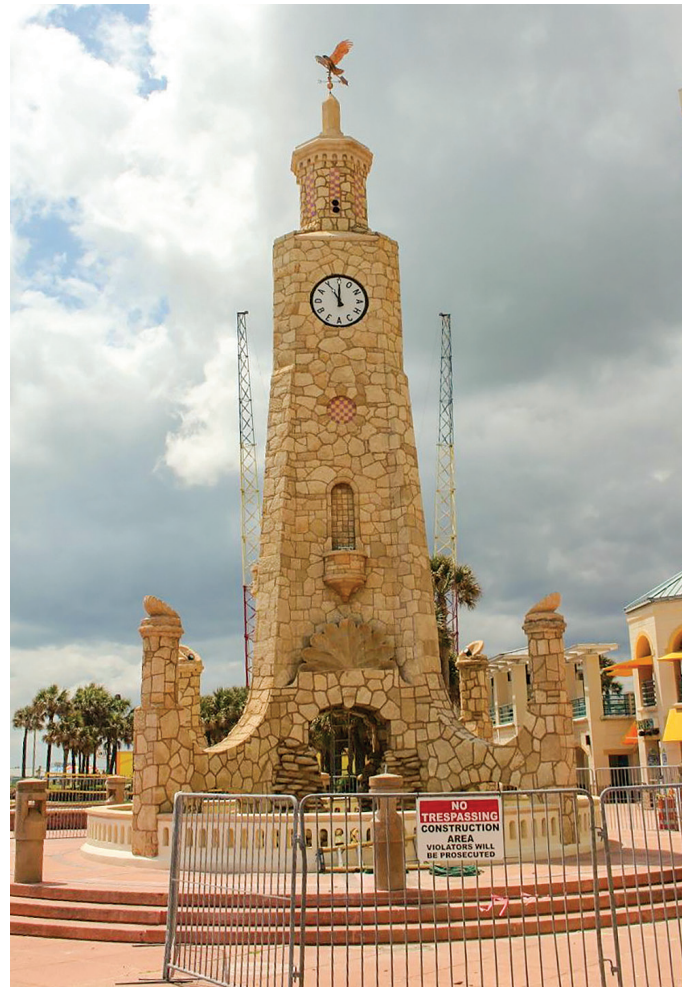
Figure 14. The restoration nearing completion. PHOTOGRAPHED BY RANDY JAYE ON JUNE 10, 2016.
